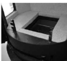
Fit 2 x steel pins in upper holes, fit baffle plate below pins fitted and resting on rear brick. Fit 2 x more steel pins to support baffle plate.
