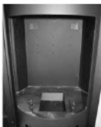
Place rear brick and side bricks in position making sure side brick fits behind location lugs at top of side windows.
