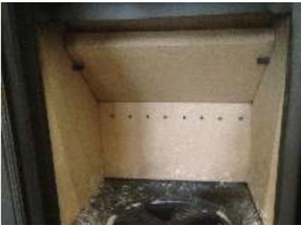
Remove lower baffle brick, slide baffle plate forward, then allow rear of baffle to drop down until baffle is vertical turn baffle and remove from chamber.
