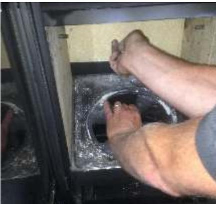
Remove base grate. Slide up rear brick 15cm, lift out grate tilting rear section upwards until front of grate is lifted out of retaining section. Turn grate sideways and remove from chamber. Lower rear brick down so it rests on base.
